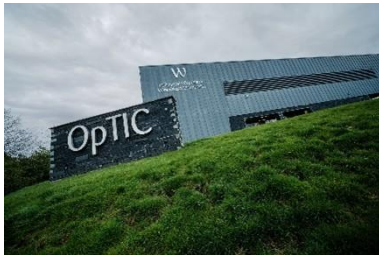
Wrexham University OpTIC Centre, St Asaph
